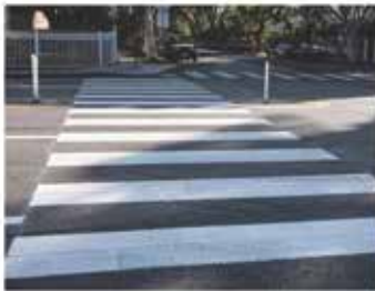
PIANO KEY CROSSWALK
