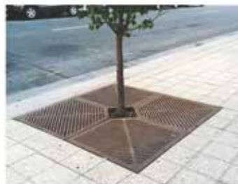
STREET TREE IN GRATE
